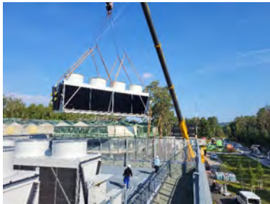
Figure 2.1: Addition of a re-cooling system on the roof of the technology center of the Faculty of Natural Sciences.
