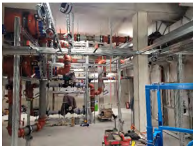
Figure 2.3: Preparations for the cooling system of the new parallel compute cluster, summer 2021.
